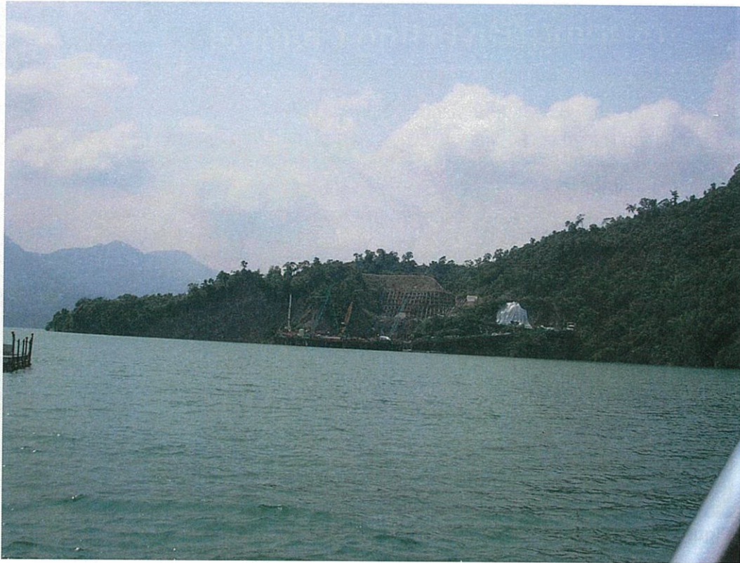
Photo 6. - Portal to Sluicing Tunnel
