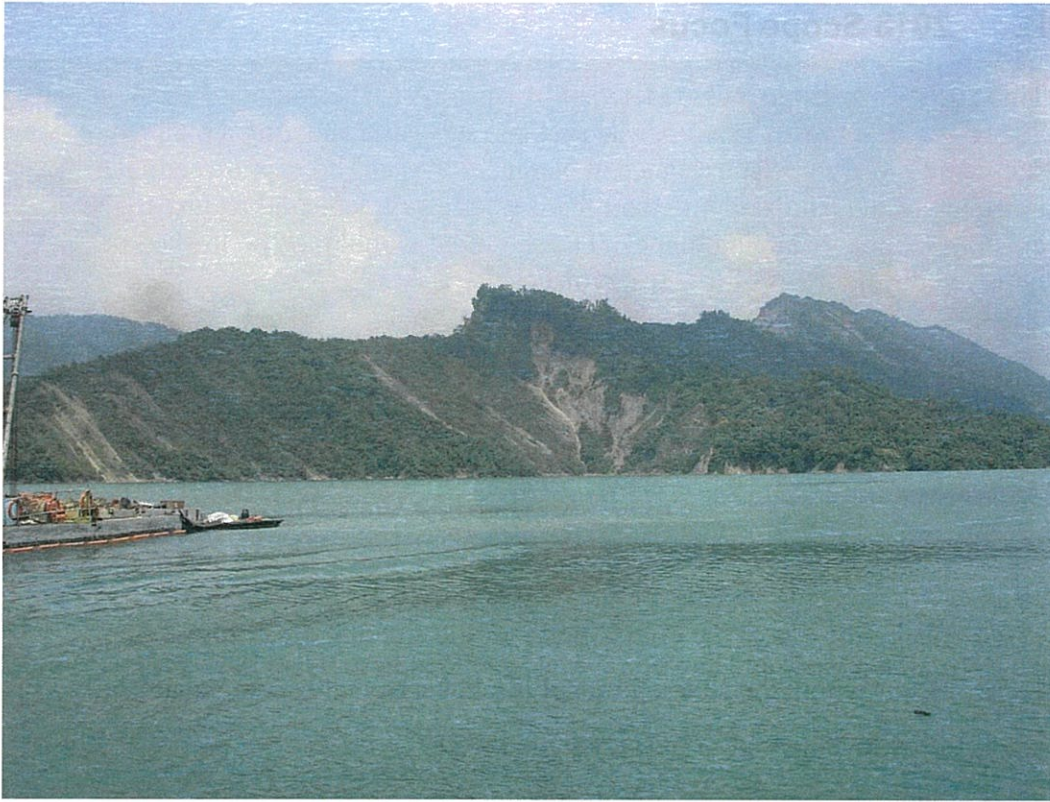
Photo 5. - Adverse Geology Related to Portal for Sluicing Tunnel
