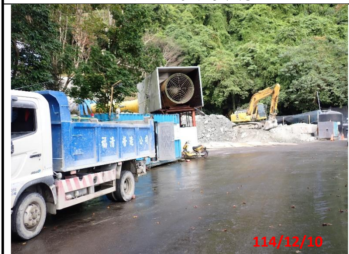
隧道進口處周邊環境
