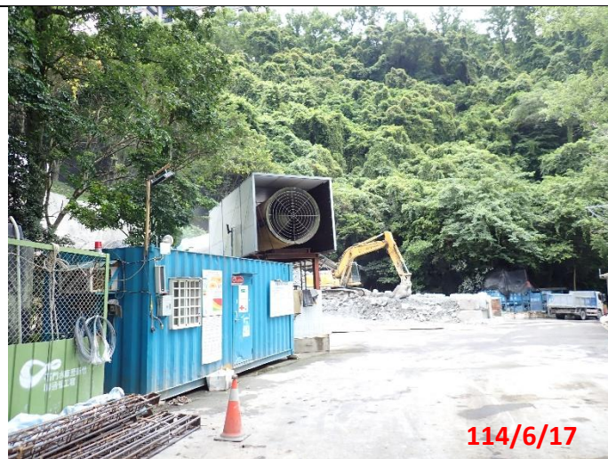
隧道進口處周邊環境
