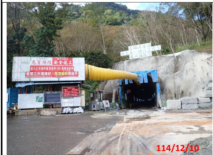
隧道進口處周邊環境
