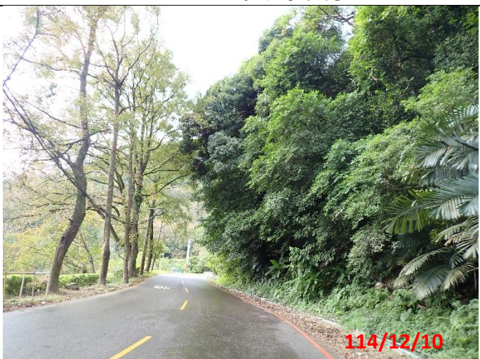
隧道進口處周邊環境
