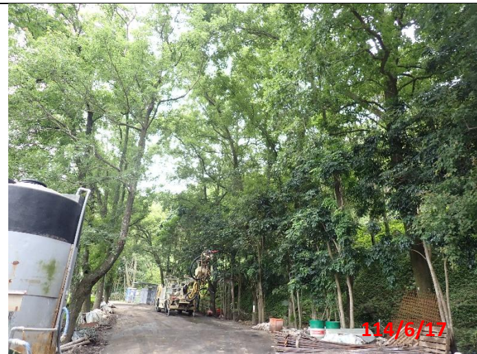
隧道進口處周邊環境
