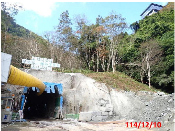
隧道進口處周邊環境
