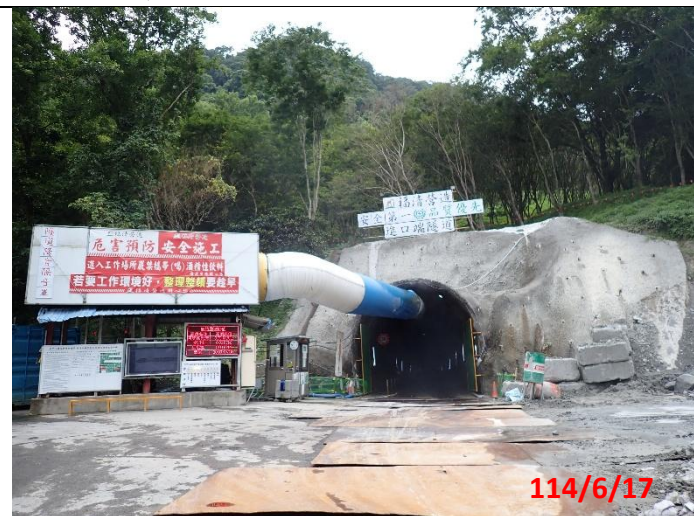
隧道進口處周邊環境
