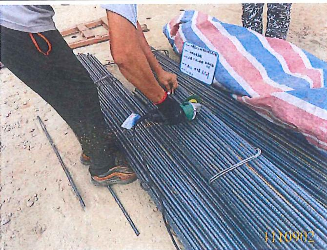
SD280W D13 鋼筋取樣
