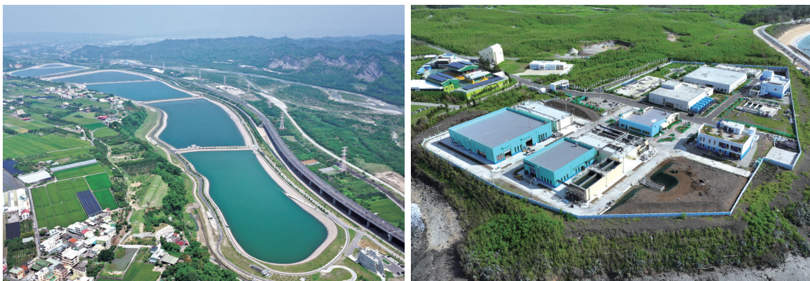
(Left) Niaozeitan Artificial Lake. (Right) Magong 6000-ton Desalination Plant.
