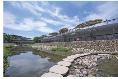
Starting by removing concrete slabs from Yunlin River, the government aims to restore vibrant ecosystems and transform the area into an important site for public water recreation.
