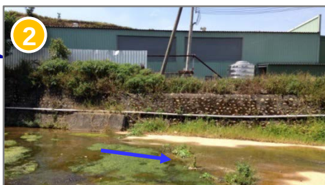
南勢坑溪0K+274下游左岸附掛管線取水
