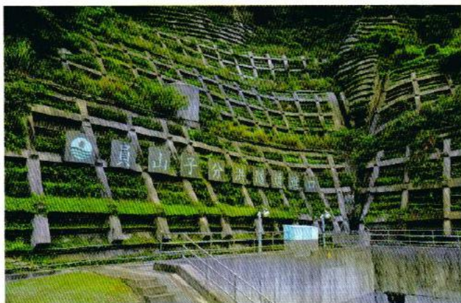
隧道進口上方邊坡
