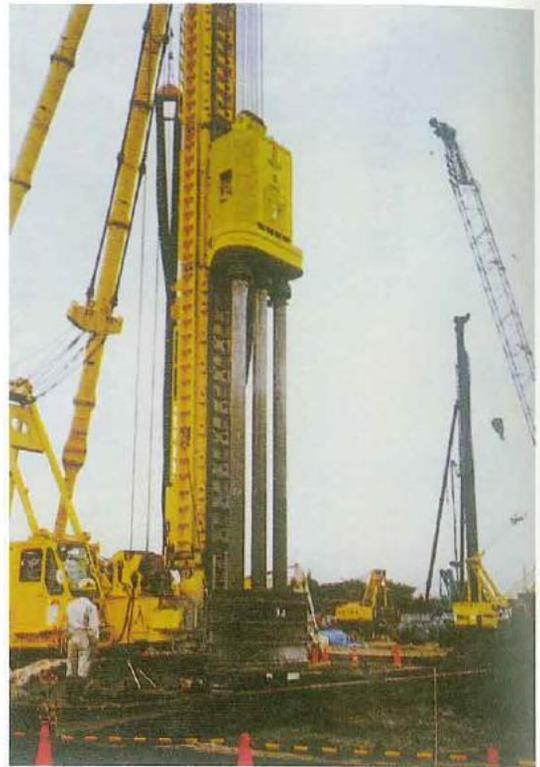
SMW ( Soil-Cement Mixing Wall ) 摻土水泥連續壁
