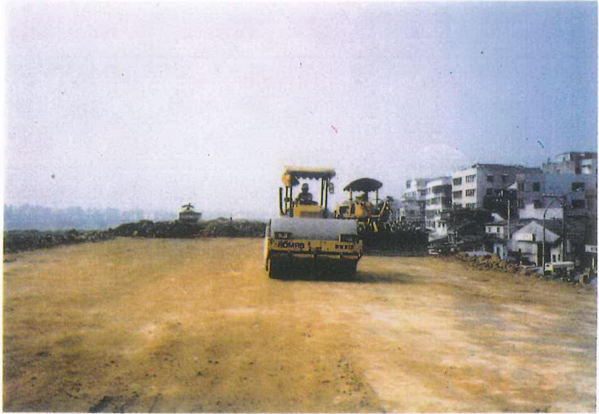
堤防填方碾壓
