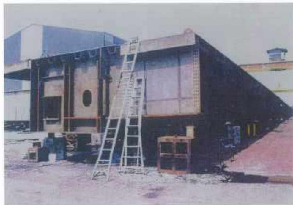
鋼橋在工廠預裝，檢查後運至工地吊裝
