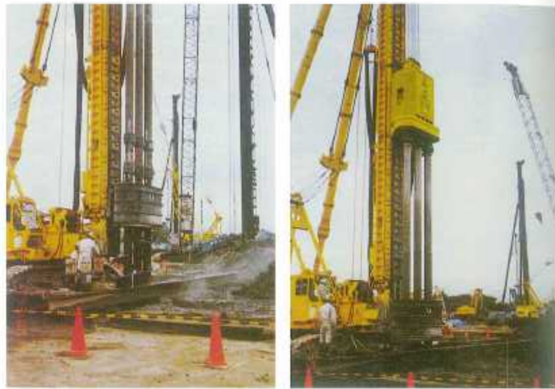
SMW (Soil-Cement Mixing Wall) 掺土水泥連續壁
