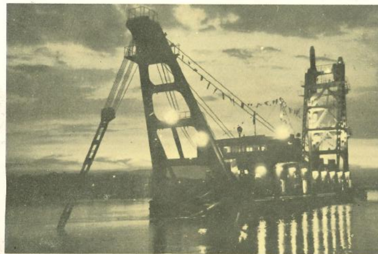
大型挖泥船漏夜趕工 2,000 HP dredger in operating at night.
