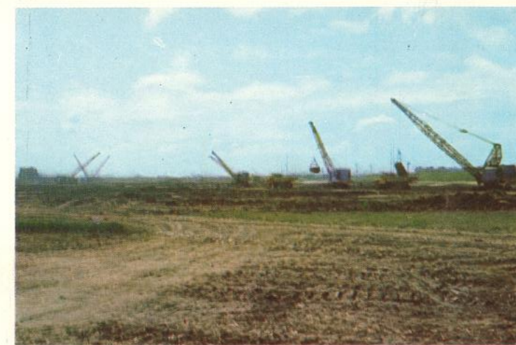
新河道開挖之陸上機具 Land equipments in operating.
