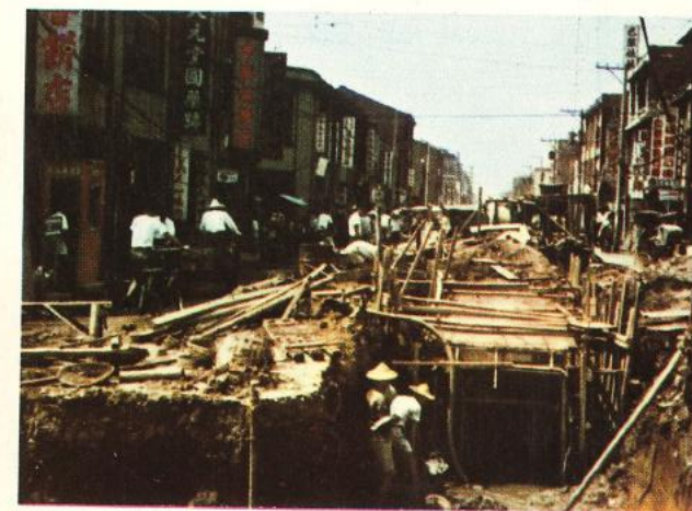
台北市下水道施工情形 Storm sewerage being constructed in Taipei city.
