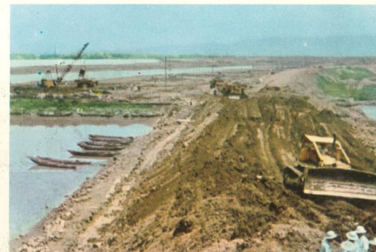
堤防填築之重機具作業 Embanking with heavy equipments.
