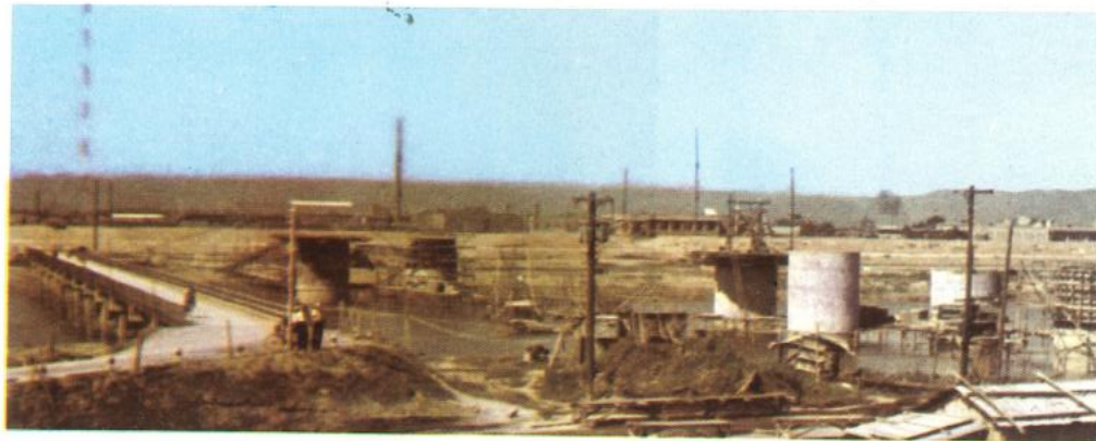
士林中正橋改建施工與臨時便橋 The piers of Chung-Cheng Bridge, located at Shih-Lin, are being constructed, and a temporary bridge beside.
