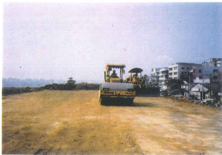
堤防填方碾壓
