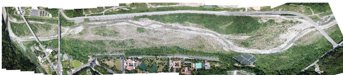
(A)施工前空拍影像(109/07/03)
