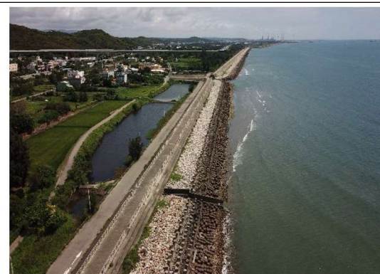
說明：新埔堤防現況(109/06/12)
