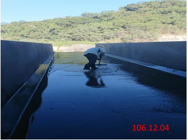
A worker in a white protective suit and mask is crouching on a wet, dark concrete floor, using a red hose to spray water onto the surface. The floor is now clean and dark. A large concrete wall is visible in the background.<br>106.12.04                                      | 導流槽清洗去除青苔。 |
