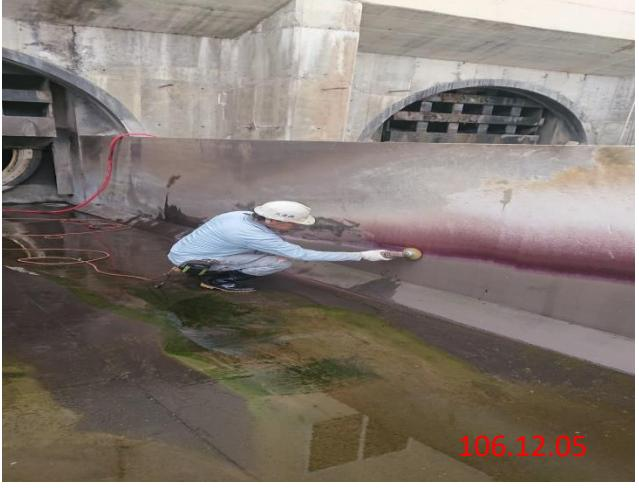
A worker in a light blue long-sleeved shirt and a white hard hat is crouching on a wet, dark concrete floor, using a yellow power tool to grind the surface. A red hose is connected to the tool. A large circular concrete structure is visible in the background.<br>106.12.05 | 導流槽除鏽研磨中。  |
