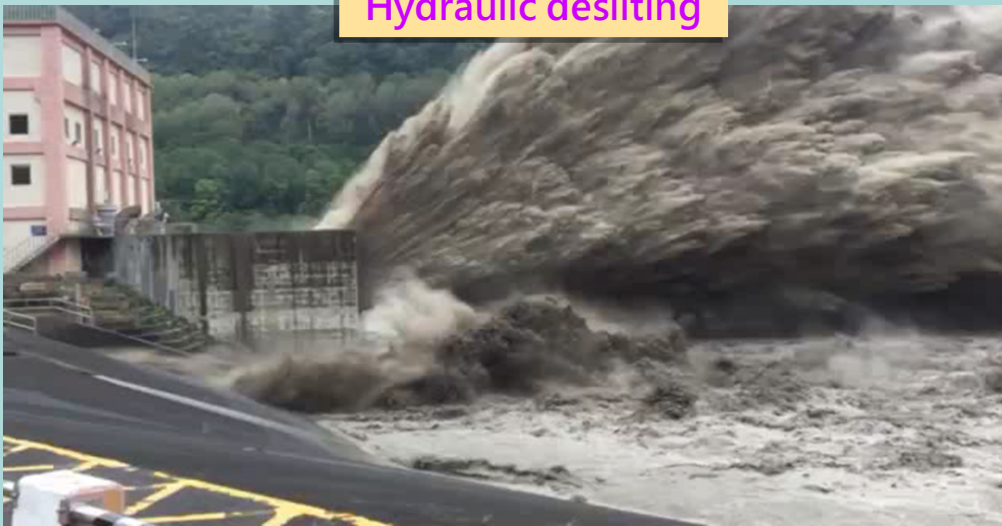
Hydraulic desilting
