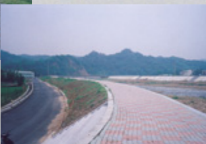
▲Siaoli River Sihzuowu Dike Reconstruction Project
