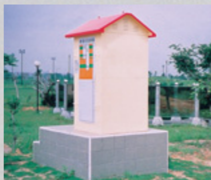
▲Hsin Chu Science-Based Industrial Park Groundwater Observation Well
