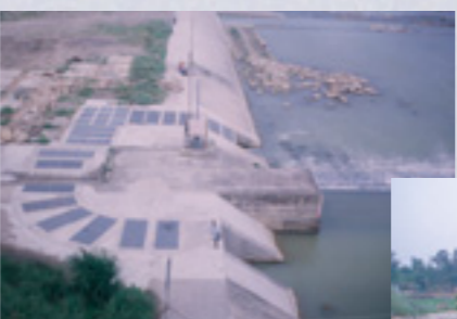
▲Toucian River Longen Weir Fish Ladder Project
