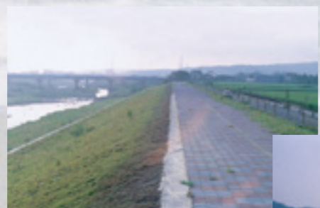
▲Fongshan River Fangliu Dike Reconstruction Project
