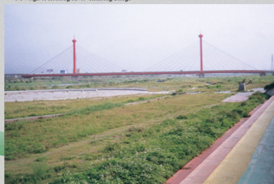
▼New sign of Huolong River -Hsintong Bridge
