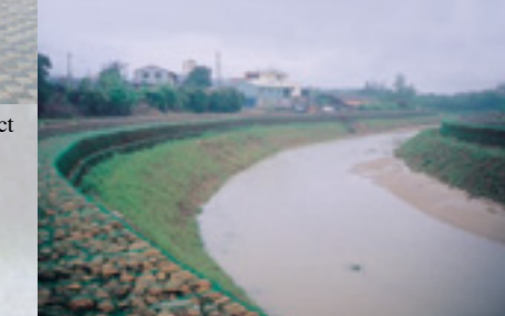
▲Yangang River Nan-ai Section Drainage Project.
