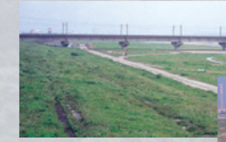
▲Toucian River Douulun Dike Construction
