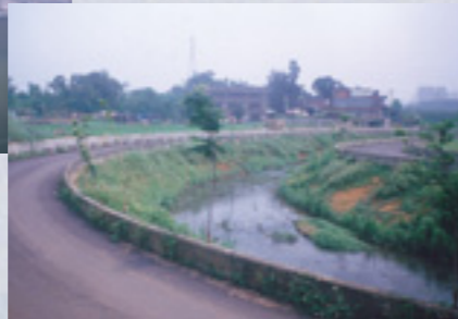
▲Kezihhu River Embankment Project
